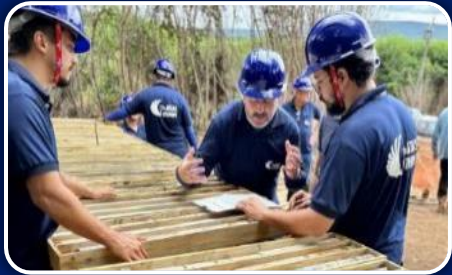
Permitted Project with Clear Path to Production
